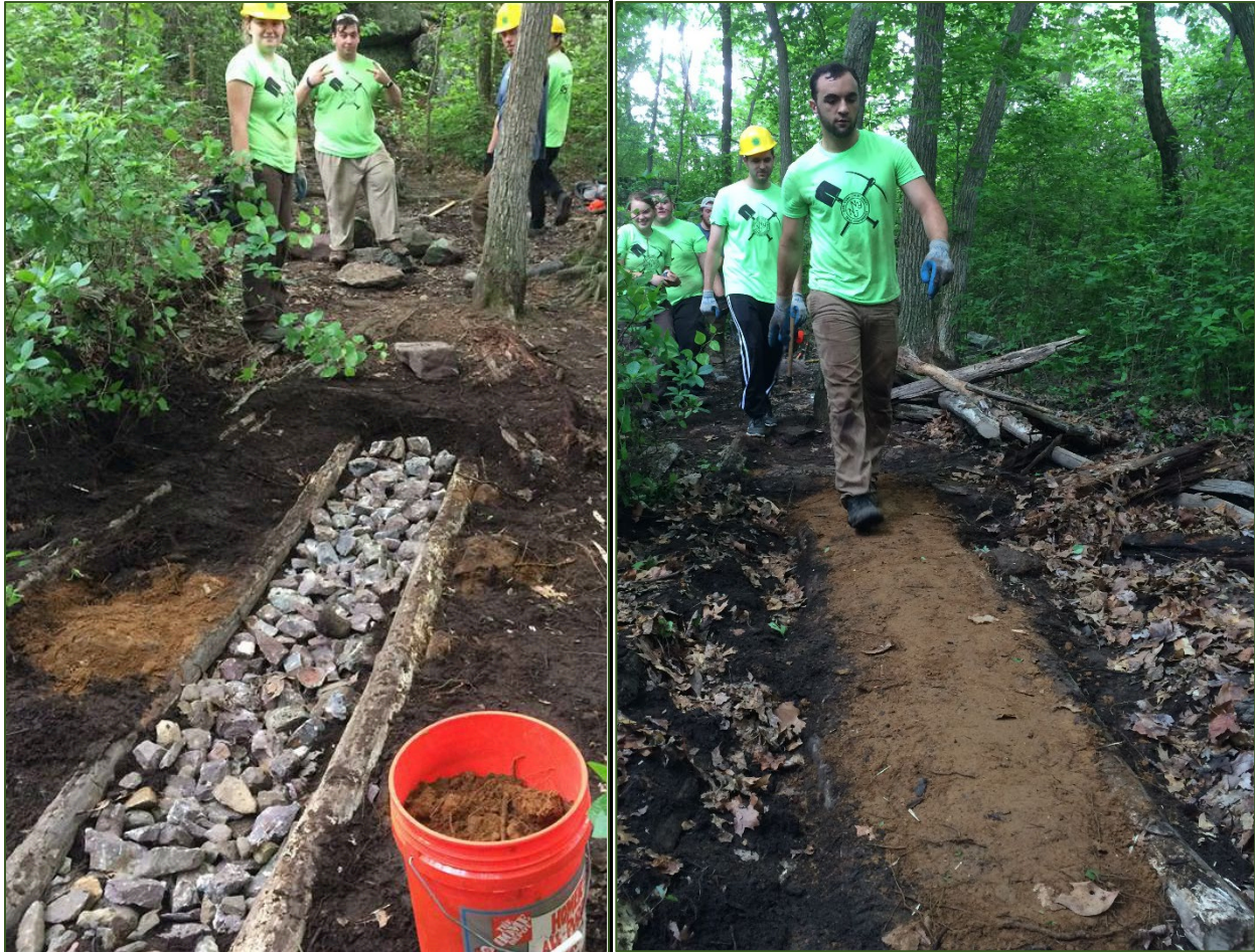
Timber turnpike after crush fill, and after mineral soil surfacing.
