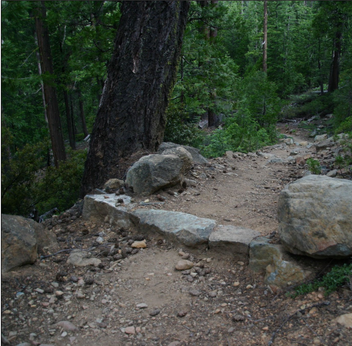
A stone waterbar, with the runoff drain visible on the left.
