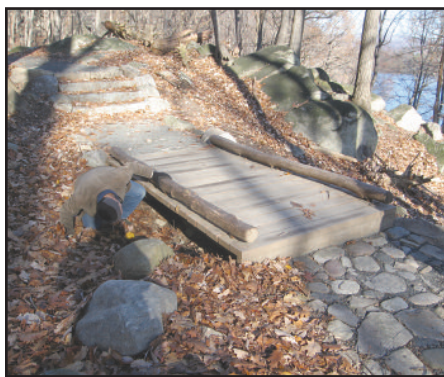
Paving and Bridge
